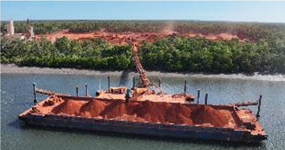
Figure 37: Barge loading at Skardon River port
